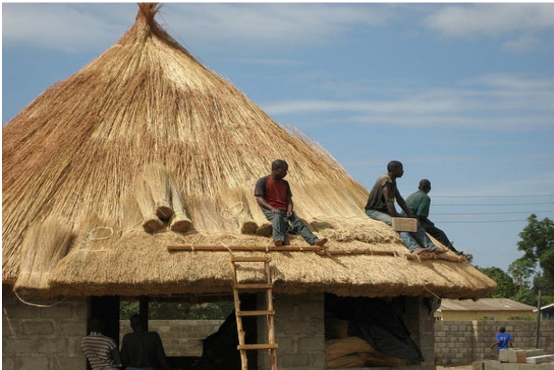
Thatching Arts building roof
